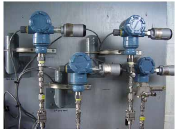
Rosemount 2051 Pressure Transmitters with Smart Wireless THUM Adapter
