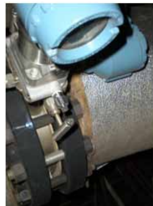
Figure 2: Compact Annubar Flowmeter installed between two raised-face flanges.
