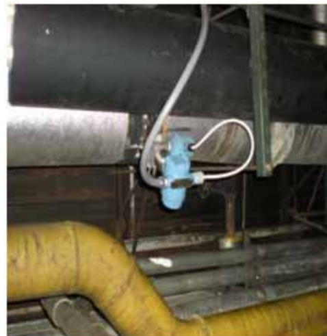
Figure 1. Rosemount 3051SFC Compact Annubar Flowmeter installation
