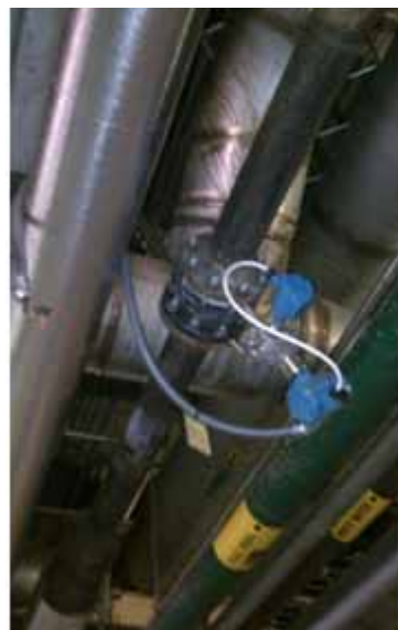
Figure 1: The Compact Annubar Flowmeter installed between two raised-face flanges.
