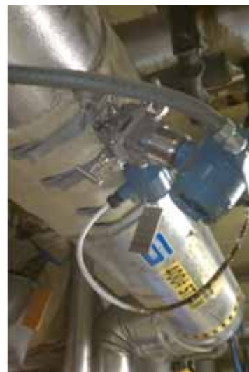
Figure 1: The Compact Annubar included integral temperature which provided a more accurate measurement and allowed the machinery to run more efficiently.
