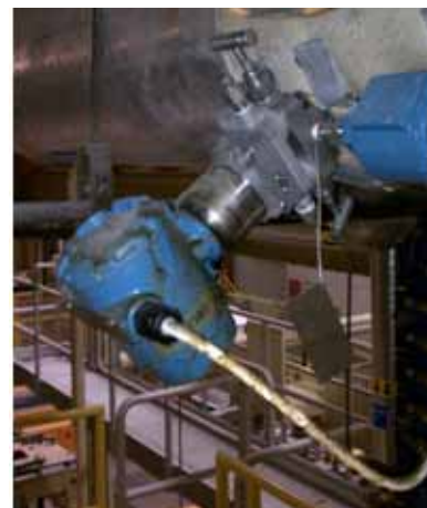
Figure 2: Compact Annubar Flowmeter installed between two raised face flanges.
