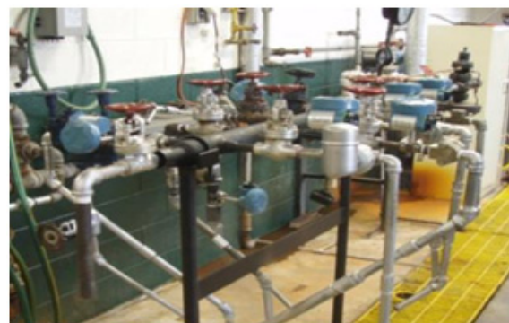
Rosemount 708 Wireless Acoustic Transmitters provide non-intrusive, continuous on-line steam trap monitoring.
