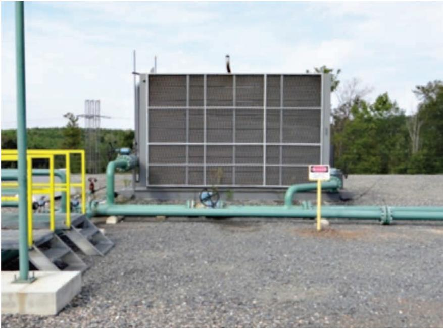
Gas-driven cooler reduces temperature to an acceptable range (Fig. 4).
