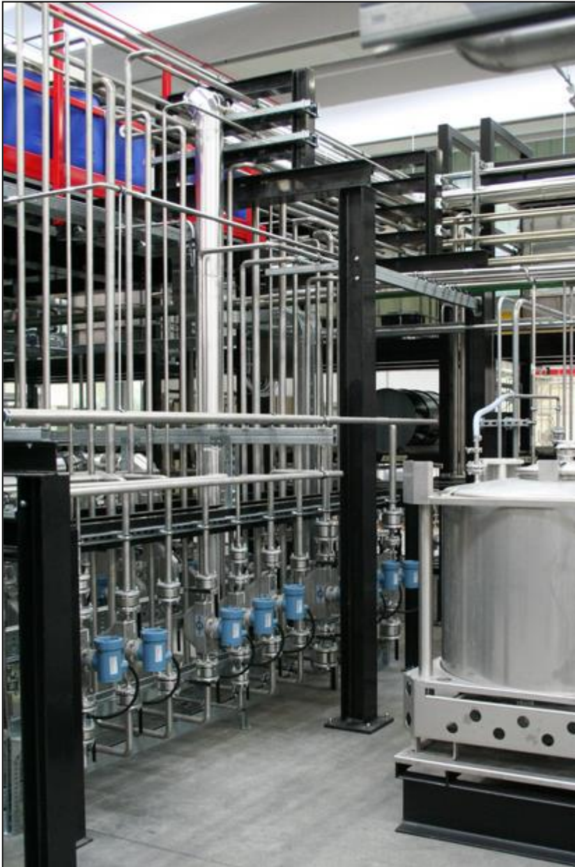
1/ A VIEW OF THE KIIAN DIGITAL PLANT IN NOVEDRATE
