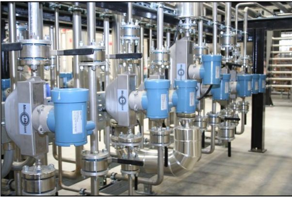
3/ THE MICRO MOTION MASS FLOW METERS PROVIDED BY EMERSON PROCESS MANAGEMENT
