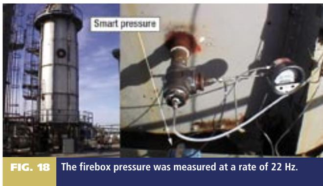
**FIG. 18** The firebox pressure was measured at a rate of 22 Hz.
