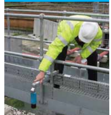
3107 Pumping station level
