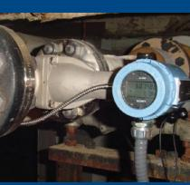
A chemical processing company installed Micro Motion meters on three chlorine lines feeding each unit—immediately reducing seven potential leak points per line and tripling accuracy.
