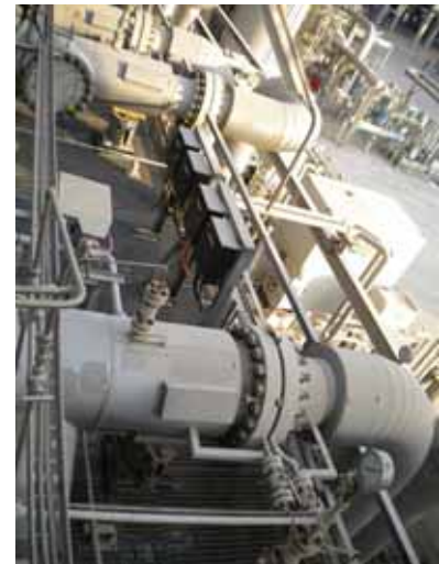
Rosemount 1595 Conditioning Orifice Plate
