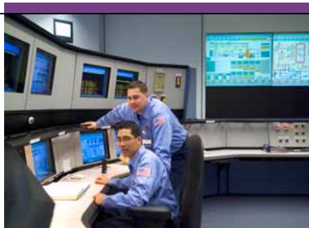
Con Edison's operators learn how to efficiently operate the ERRP Ovation control system, as shown in the control room photos above and below, by using a customized high-fidelity Ovation Simulator.
