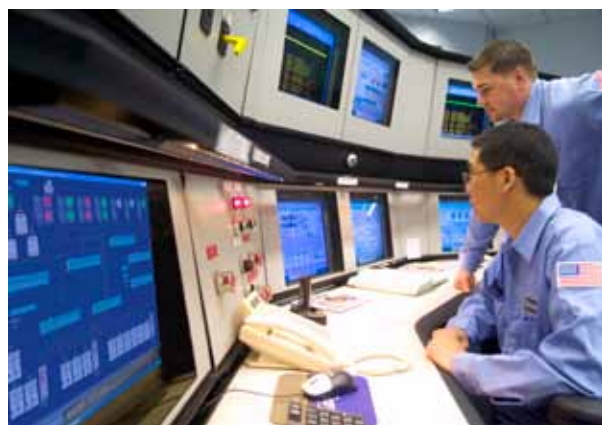
Con Edison's operators learn how to efficiently operate the ERRP Ovation control system, as shown in the control room photos above and below, by using a customized high-fidelity Ovation Simulator.
