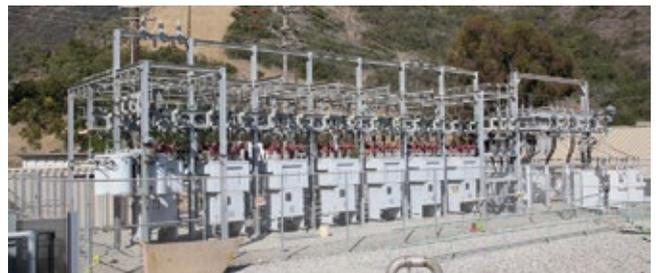
**3. SCADA technology** provided by Emerson Process Management helps maintain a stable grid voltage. Photo is of Catalina's 12-kV switchyard
