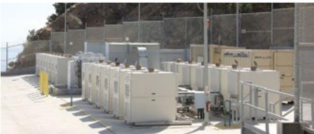
**2. Microturbines** supplied by Capstone Turbine Corp provide the flexible generating capability required on Catalina Island
