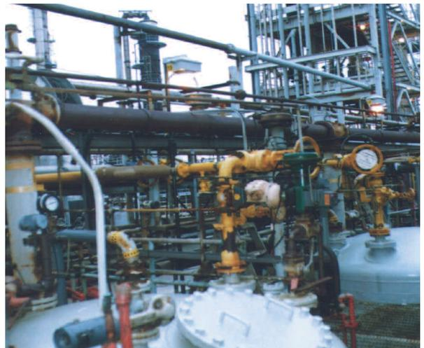
*The Micro Motion meter was installed horizontally to prevent trapping of liquid and/or gas.*
