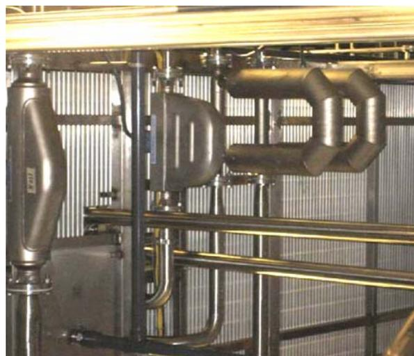
Figure 3 A Family Affair – Micro Motion F, R and CMF (ELITE) Direct Connect Meters in Beverage Blending Plant
