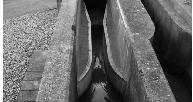
Venturi flume: BS3680 Part 4C / ISO 4359
