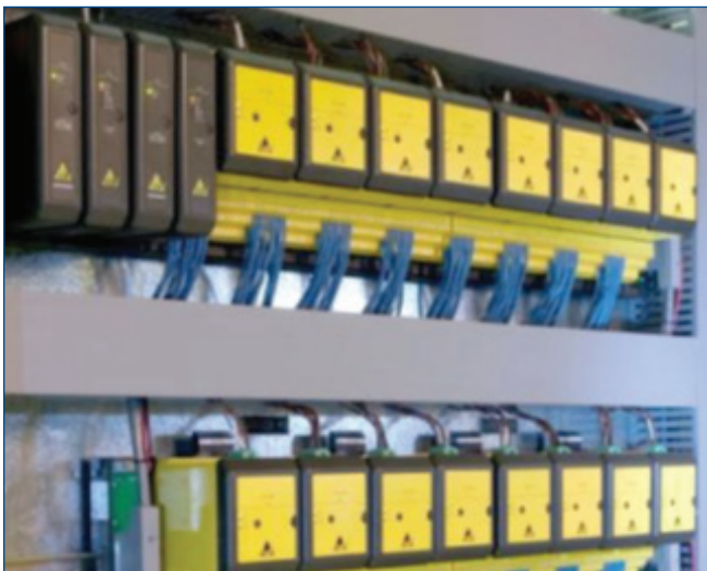
DeltaV SIS logic solvers mounted horizontally.
