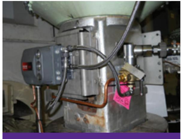
*AFTER*—Since the FIELDVUE™ digital valve controllers and high-capacity solenoids were installed, the plant has experienced no trips. Connected to the system via a HART® Interface Module, the FIELDVUE instruments provide data about valve performance and alert operators of any problems.
