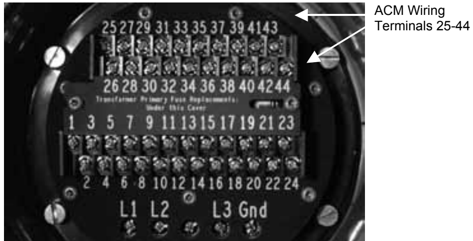
Figure 3-10 ACM Wiring Connections
