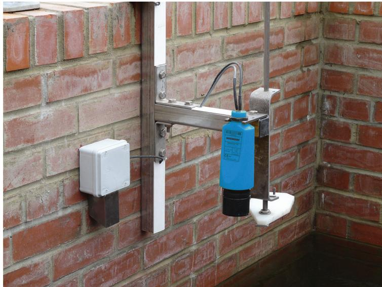
Figure 3-7. Enclosed or partially covered flume chamber arrangement
