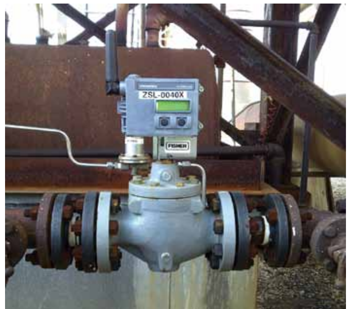
Fisher Type EZR with Topworx Type 4310 Wireless Position Monitor
