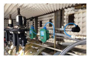
Figure 1: Axial Flow Pressure Regulators equipped with RAF system
