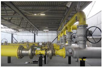
Figure 3: Axial Flow Pressure Regulators equipped with RAF system
