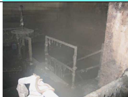
A view of the conditions of the sewage pumping station.
