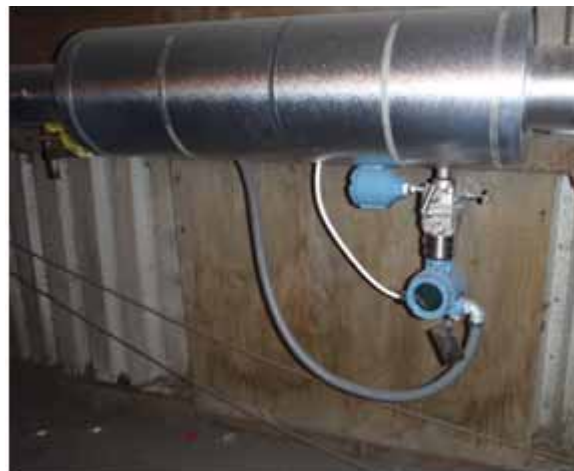
Figure 1. Rosemount Compact Annubar Flowmeter installation.
