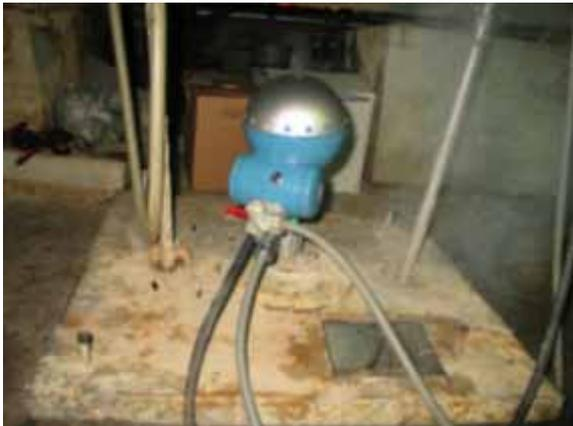
The 5600 was installed with a second analog output line so that signal strength could be monitored.
