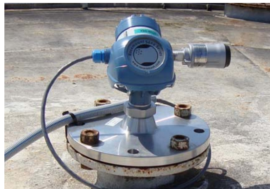
Rosemount 5402 non-contacting radar measurement devices with Smart Wireless THUM's were placed on large tanks and over floating roofs to automate tank level measurements and overspill protection.
