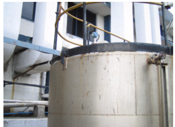
The Rosemount 3300 fit into the existing connection on the propylene glycol tank.
