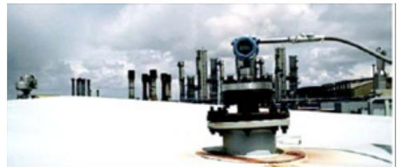
*Rosemount 3300 installed on salt water disposal tank.*
