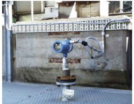
The Rosemount 3300 reliably measures level and interface in pump sump pits.
