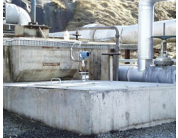
The Rosemount 3300 reliably measures level and interface in pump sump pits.
