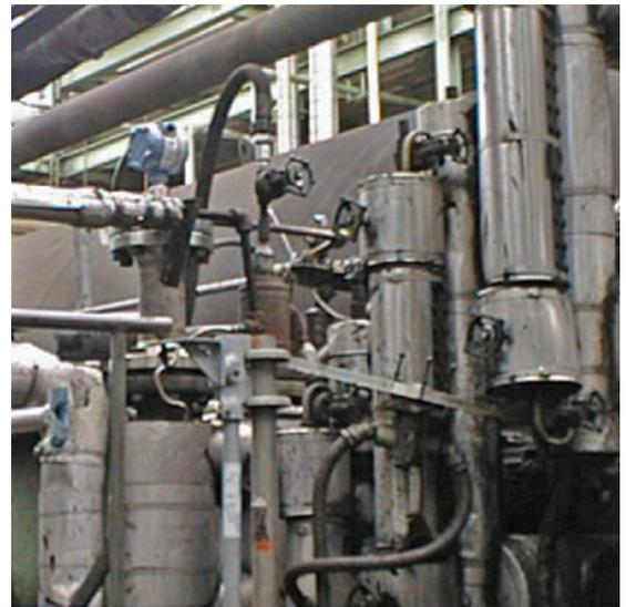
*When first installed, the 3300 was mounted next to the displacer so both devices detected the same interface.*
