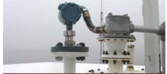
*The Rosemount 3300 Guided Wave Radar was chosen for its diagnostic capabilities and easy-to-use software tools.*
