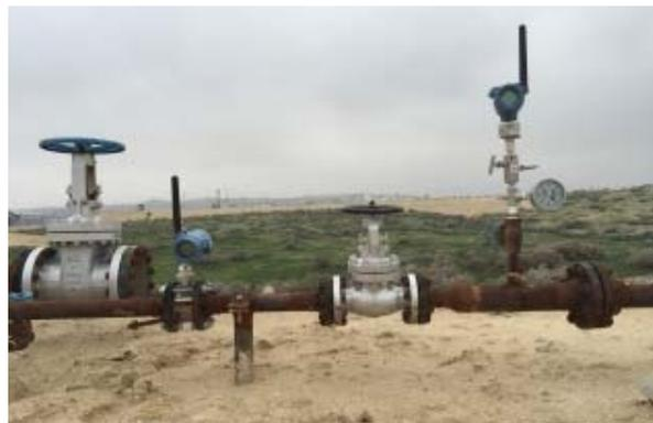
*A wireless 705 Totalizer provides flow and totalized injection volume of wastewater. A wireless 3051S provides online injection pressure to indicate stoppage.*
