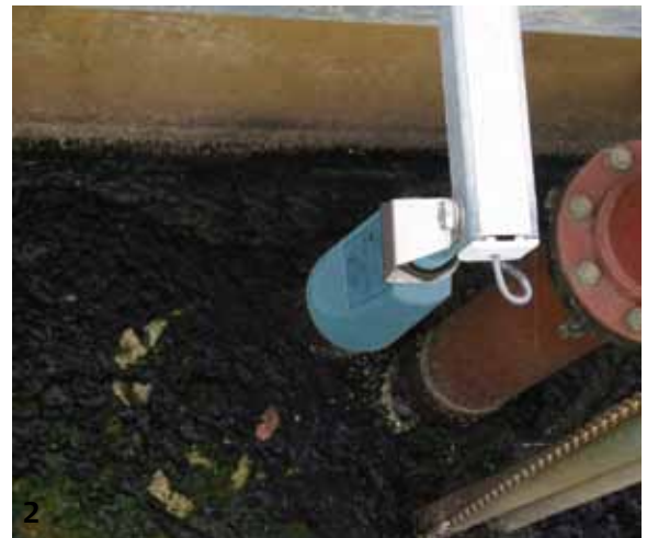
A Rosemount 3107 mounted above a wetwell.
