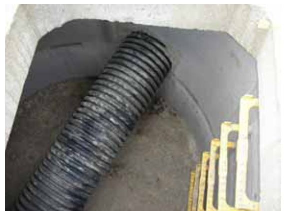
Figure 1. Manhole chamber showing original pipe running directly through the chamber
