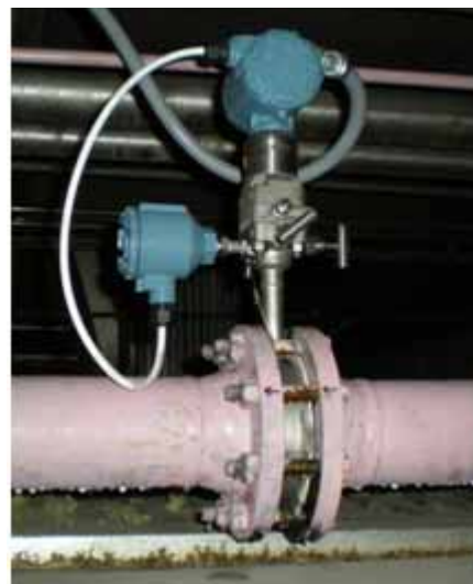
Figure 1: Rosemount 3051SFC Compact Annubar flowmeter installation between two raised face flanges.
