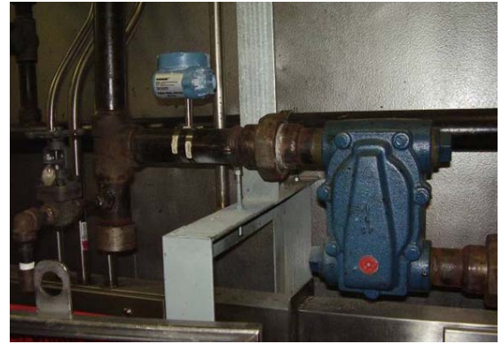
The 708 Rosemount Wireless Acoustic Transmitter features integrated sensors that mount externally to make installation fast, inexpensive, and non-intrusive to the process.
