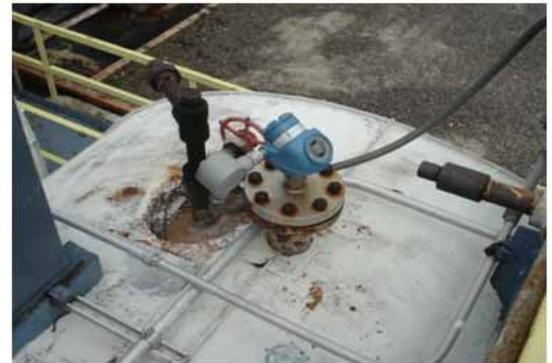
Figure 2: Rosemount 5302 Guided Wave Radar reliably measures emulsion layer on desalter vessel.
