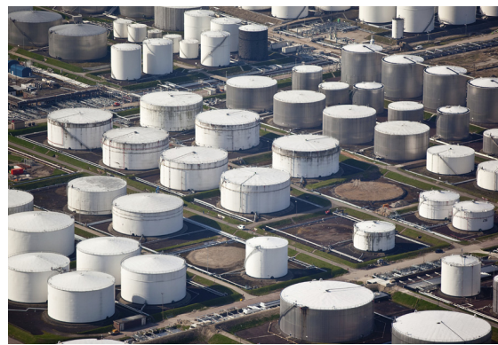
Smart wireless enables overfill protection of crude oil storage tanks during off loading from ships
