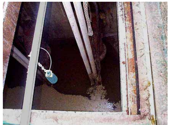
A Rosemount 3107 mounted above a wetwell.
