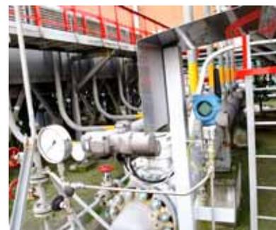
*Emerson Smart Wireless Gateways were simply added to the existing Modbus network to make data from the wireless transmitters available within the existing control system.*
