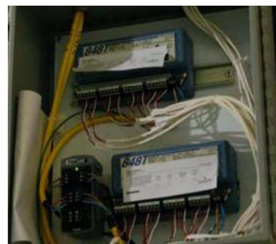
One 848T Wireless Temperature Transmitter can handle up to 4 inputs including 4-20mA, mV, Thermocouple, RTD, or ohm. The field hardened enclosures and intrinsically safe Power Module makes it ideal for this hazardous environment.
