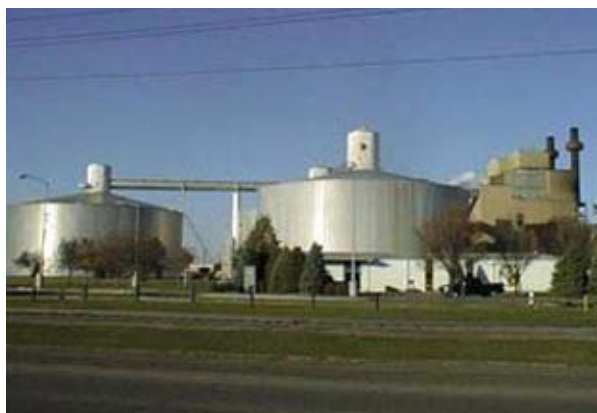
Sugar silos at ACS in EGF have a rotating bridge that made wired instrumentation impossible to implement.
