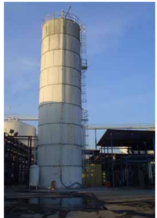
Figure 1: Diatomaceous earth is used as a wine filter and stored in this 80-ft silo.
