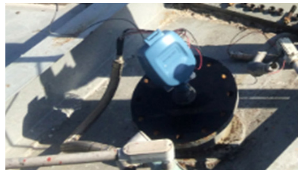
The scanner is installed using the existing connection
