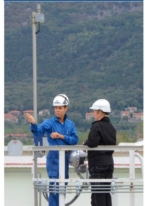
*The TankRadar Rex gauge from Emerson is connected to a Smart Wireless THUM Adapter antenna unit (mounted on the vertical pipe above the tank).*
