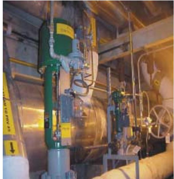
The GE application involved an inlet pressure of 50 psig at 350-degrees Fahrenheit and an outlet pressure of 10 psig at saturation. Accommodating the new valve design required some piping changes, but the Fisher Manufacturing team met the requested delivery date for the TBX units.
