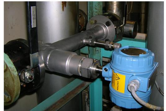
Installation of a Viscomaster meter at the Viscobooster unit (VBU) of the heater control in a ship's engine
