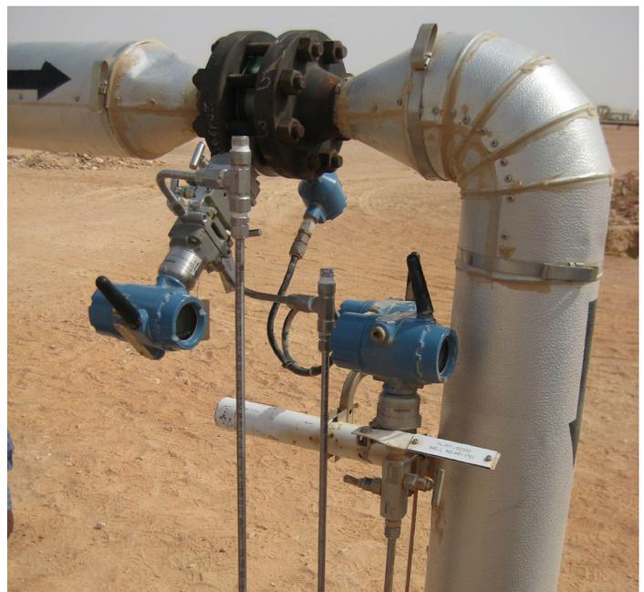
*Figure 1, wireless transmitters installed in field. This wireless installation measures steam flow injection rates in this oil and gas field by utilizing differential pressure, gauge pressure and temperature measurements. In the foreground are Rosemount 3051S differential pressure and 3051S gauge pressure transmitters. Visible in the background is the temperature connection head for the obscured Rosemount 648 wireless temperature transmitter.*
