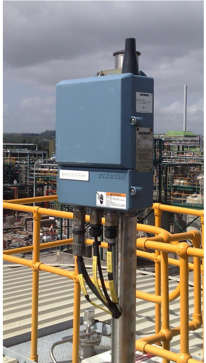
*Figure 2, gateway installed in field. This WirelessHART Gateway communicates with multiple WirelessHART field devices via a wireless mesh network, and with host systems via a hard-wired connection.*
