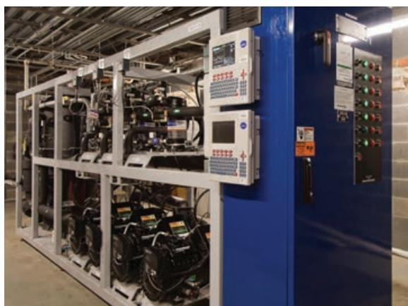
*Hillphoenix warm climate CO<sub>2</sub>-based transcritical booster system installation utilizing Emerson Climate Technologies components*
