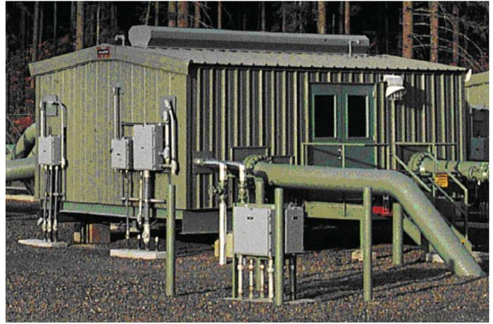
*CBM producers are putting in wellhead compression right from the start. Scroll compressors can take low suction pressure and boost it to 70-190 pounds discharge, which gives the producer more flexibility.*
