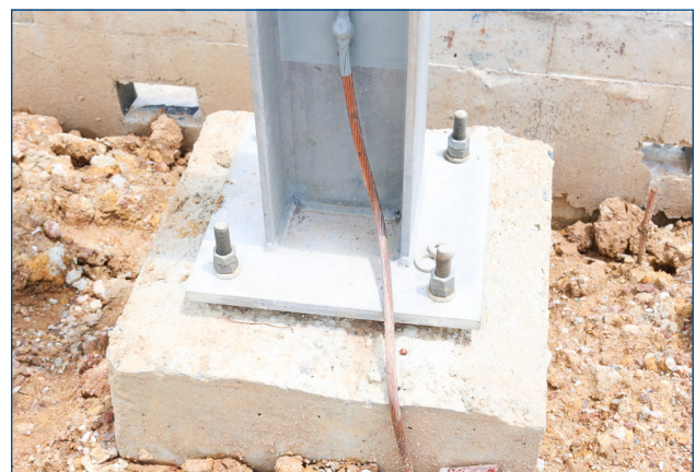
Fig. 4 Building steel used as grounding hub
