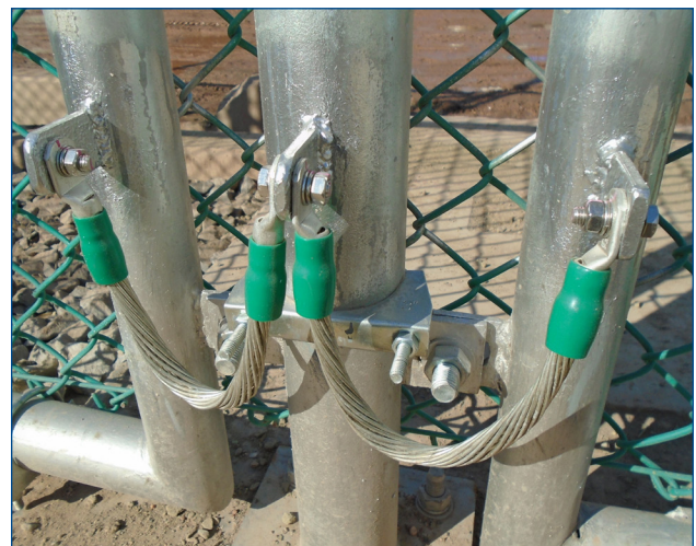
Fig. 2 Fence and gate with flexible ground connections
